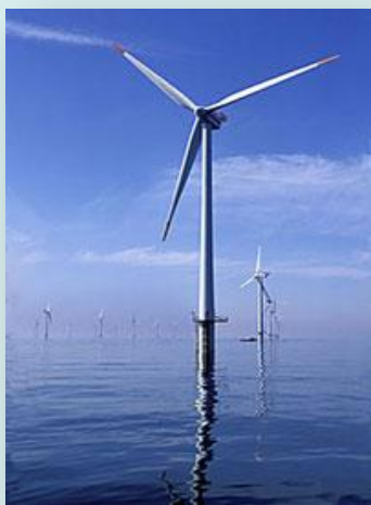
Horns Rev Offshore Wind Farm, Denmark
