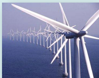
Middelgrunden Offshore Wind Farm, Denmark
